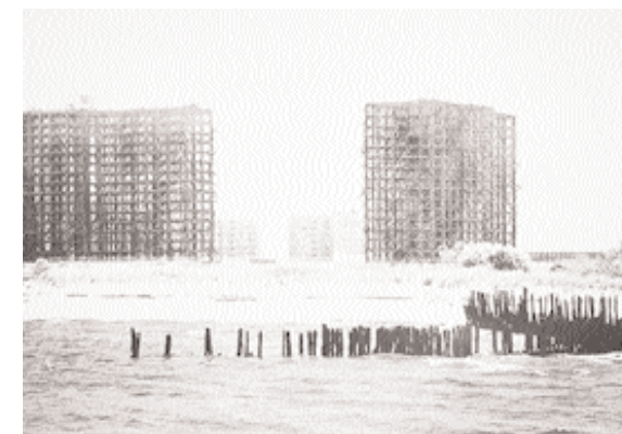
Simonds, Stanley Taukel Memorial Hanging Gardens, Breezy Point, Gateway National Park
