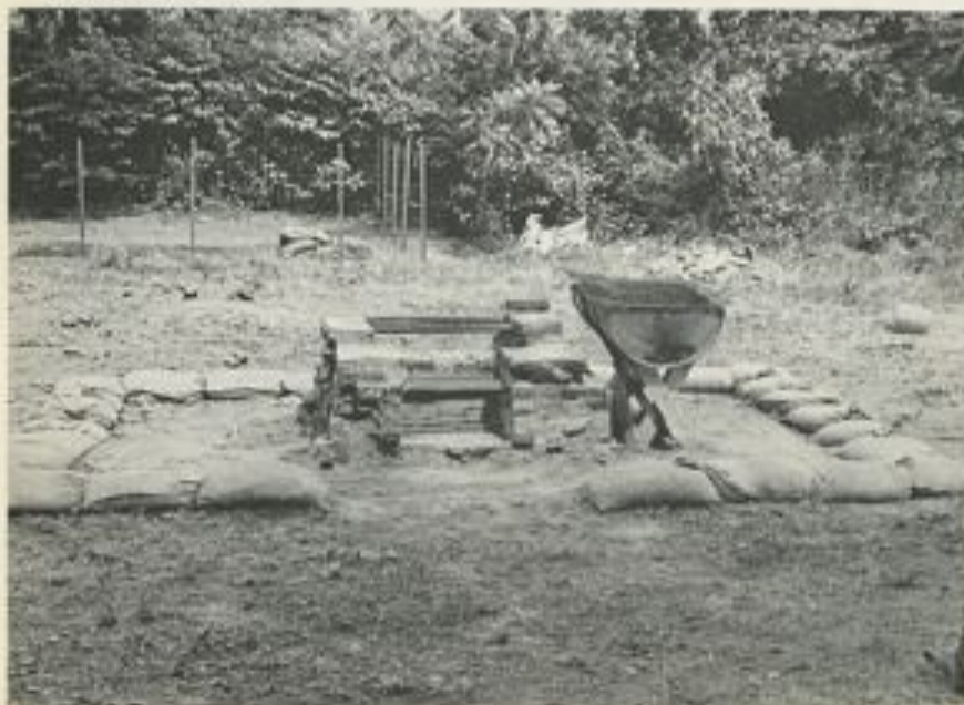
60 Completed barbecue area.
