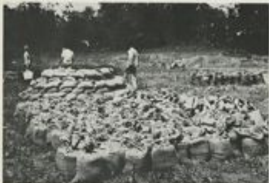
50 A day's "mess" of sandbags ready to be arranged.
